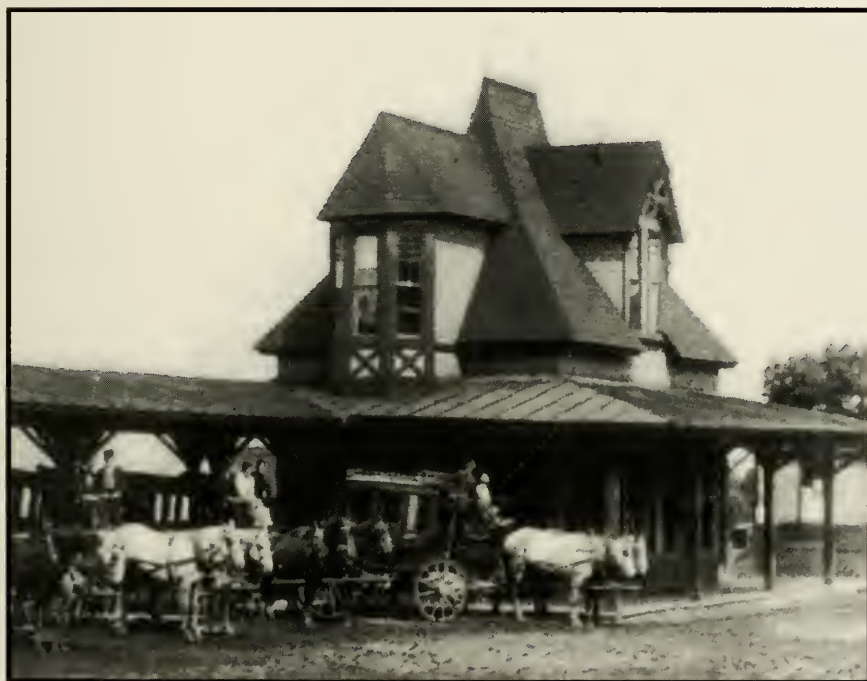
Bethlehem Train Depot ~ Birchmere Avenue ~ 1881 to Present Now A Private Home
